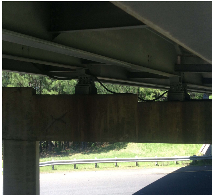
PHOTO 1 Description Bent 2 joint seal missing
